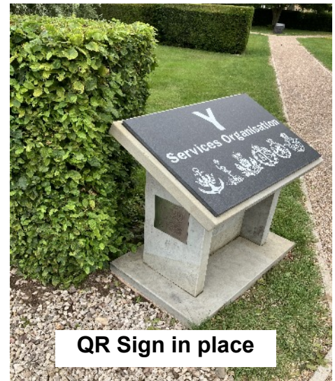
Installing the QR sign
